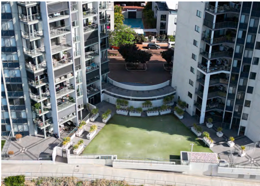
Fig. 8. Our analysis shows a disjunction between policy aspirations for green COS and the relative barrenness of constructed COS. Note: This photograph is an indicative example only as our ethics approval prevents the release data identifying the study buildings. (For interpretation of the references to colour in this figure legend, the reader is referred to the web version of this article.)
