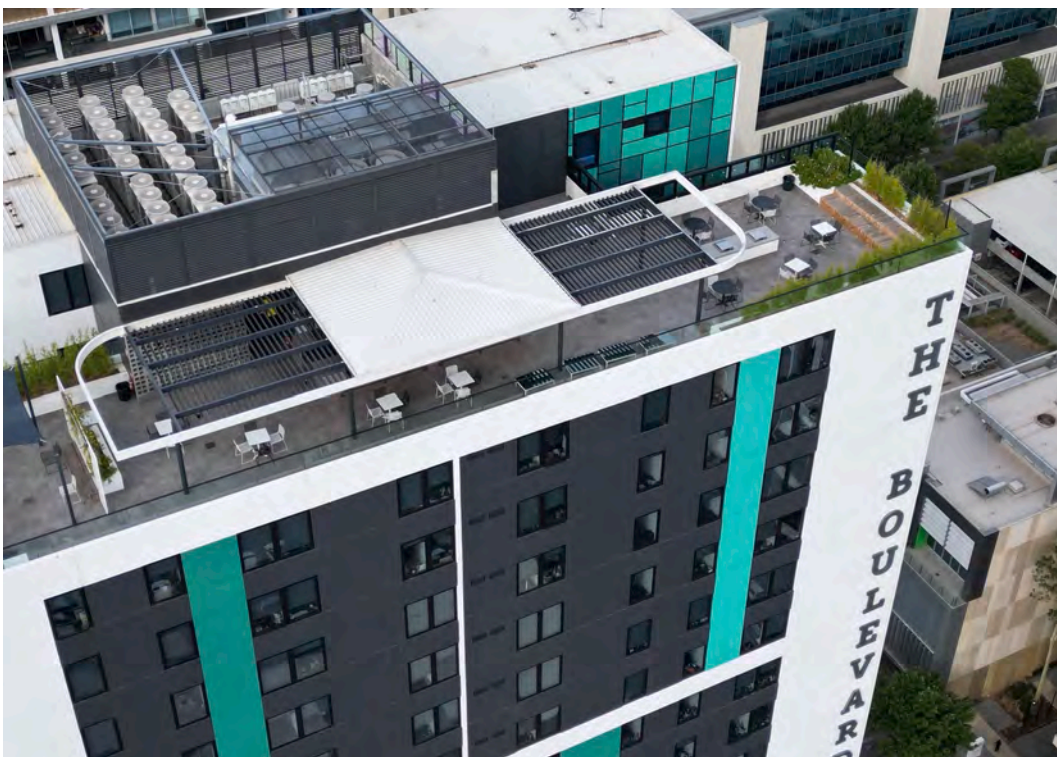
Fig. 4. COS types on building structure, such as the Roof Terrace type (pictured), also did not contain significant trees due to a lack of deep soil zones and structural constraints. Note: This photograph is an indicative example only as our ethics approval prevents the release data identifying the study buildings.
