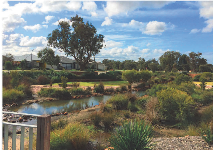
Figure 3. Living Streams. Living Streams, which arguably represent one of the most visible WSUD trademarks, are typically retrofitted drains in urbanised or urbanising areas, which aim to deliver the multiple benefits of the water cycle. This image shows a recently completed Living Stream section in the Wungong development, on Perth's south-eastern growth corridor.
